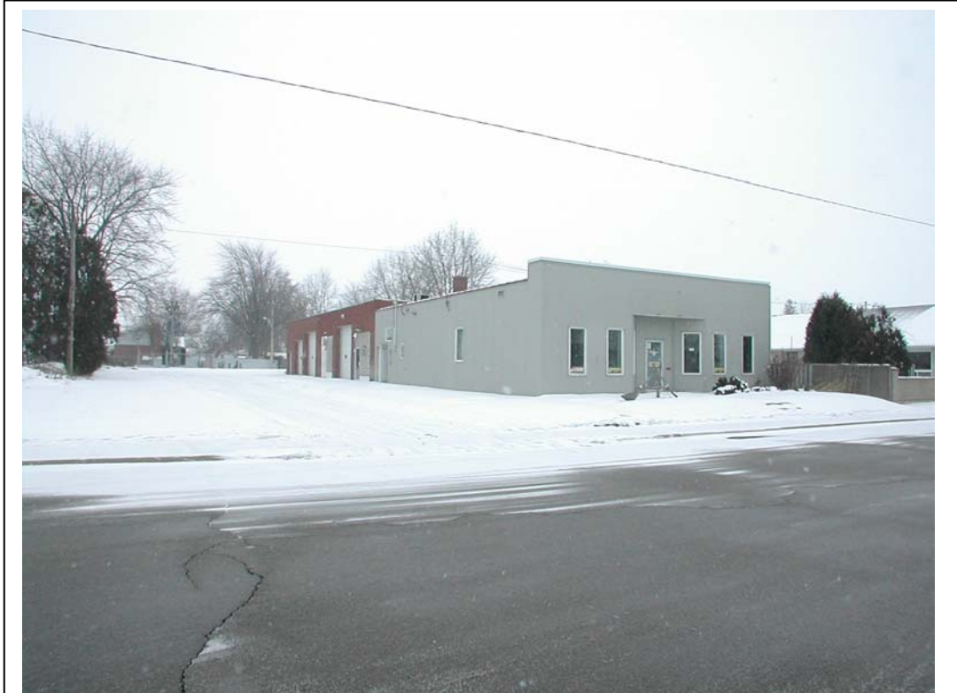
Looking south at the existing building to be converted for residential purposes
