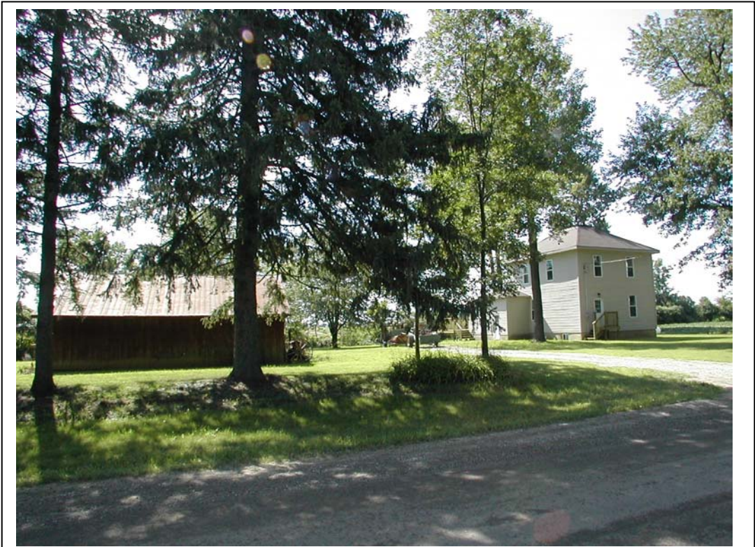
Looking southeast at the existing dwelling and outbuilding on the proposed severed parcel
