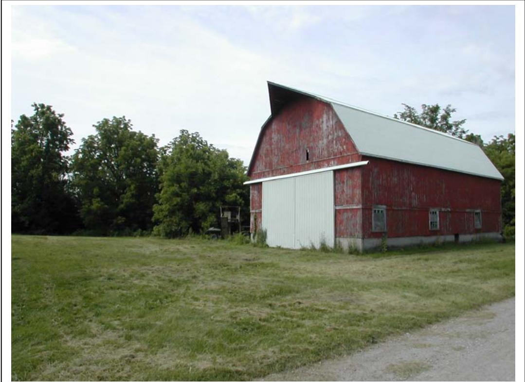
Looking southwest at one of the existing outbuildings to remain on the retained farmland
