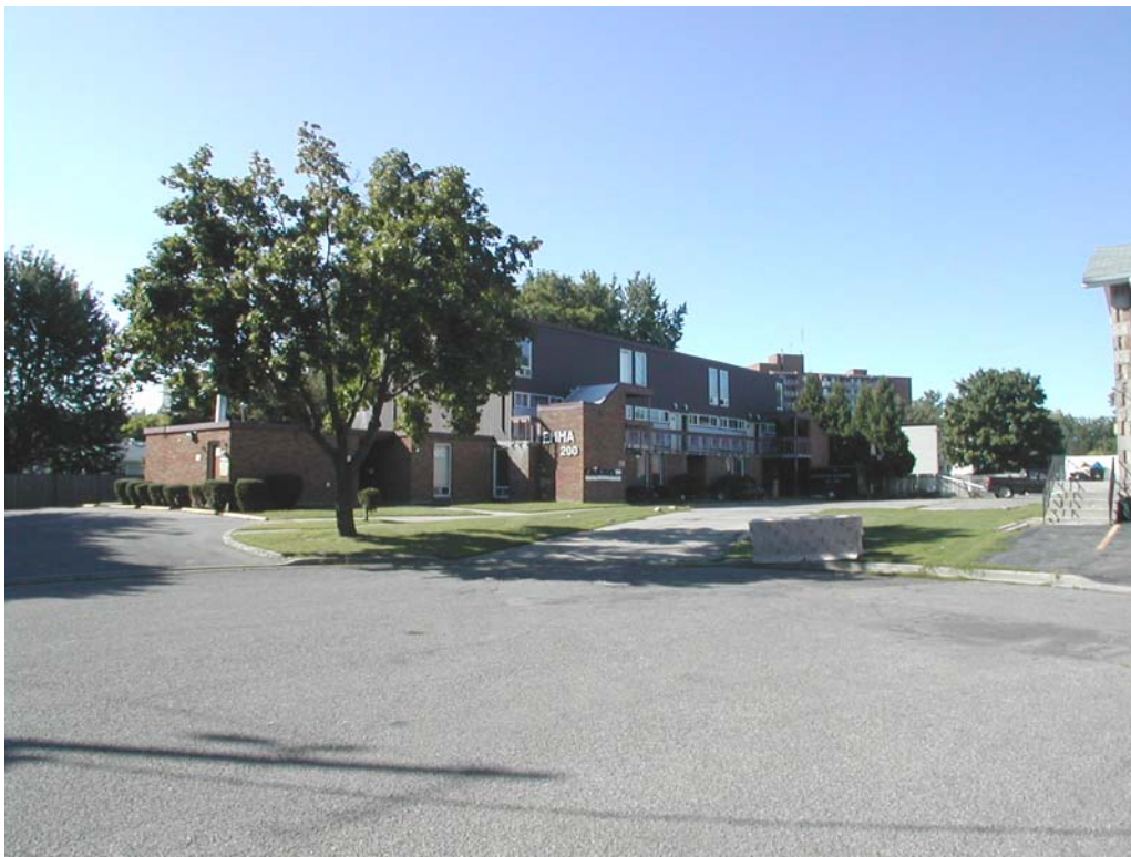
Looking southwest at the building on the subject property
