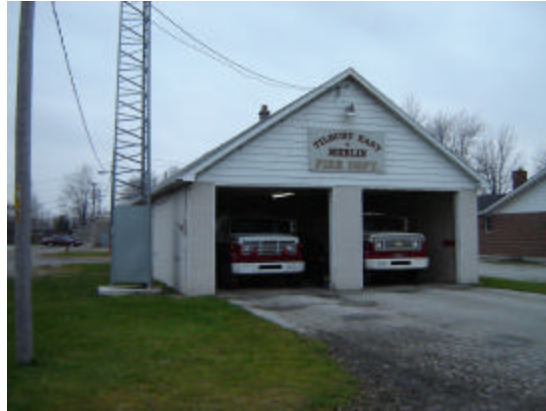
Station 17 Storage Garage
