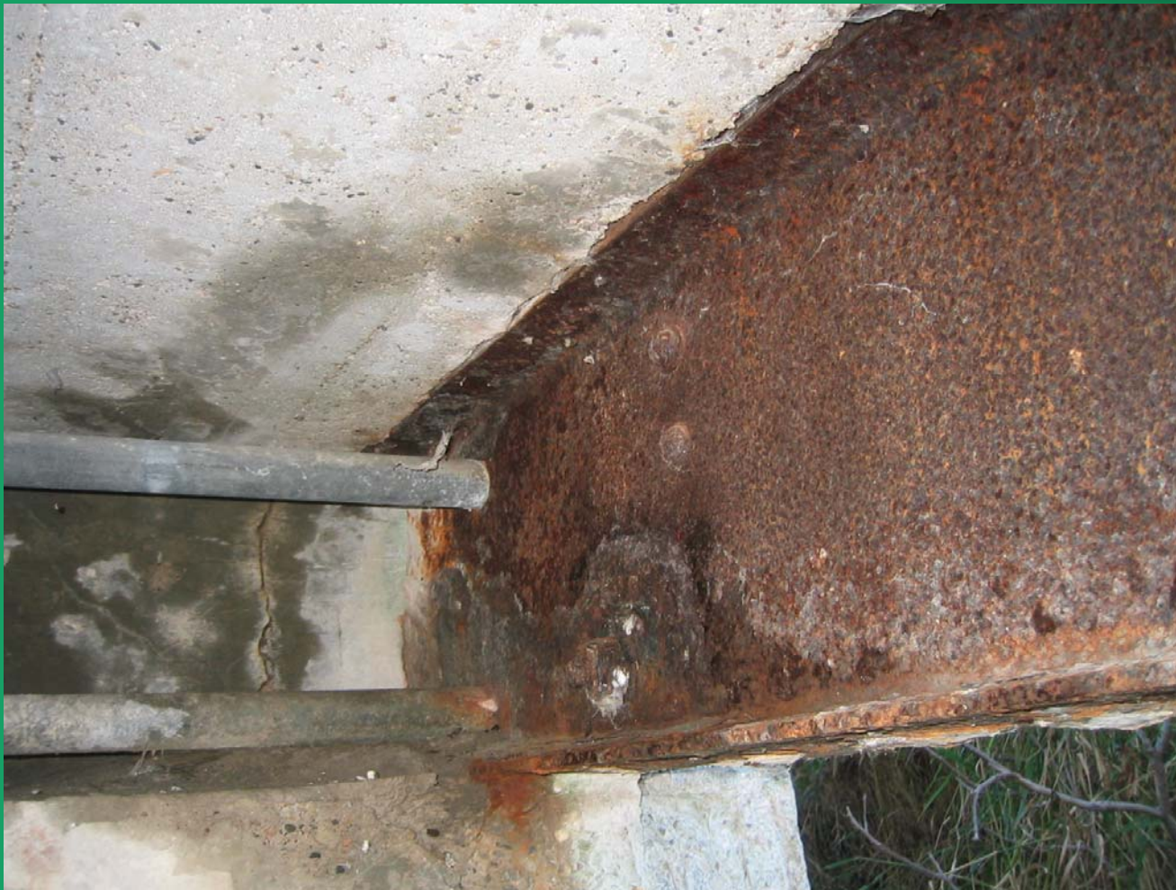
Soffit Deterioration
